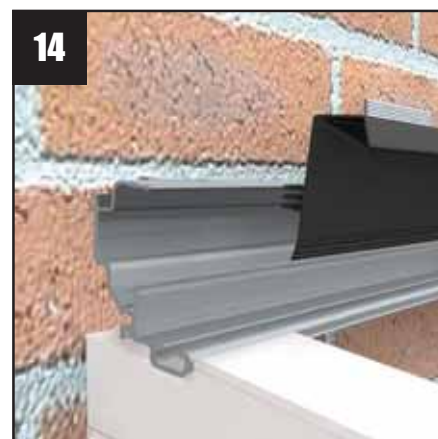
14 Fit the back and main baffle. (It is pre-cut to the external frame dimension - DO NOT CUT). You may want to grind out and fit the flashing. When fitting a starter bar attach it at 500mm centres to firring.
