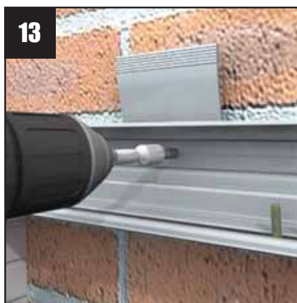
13 Systematically install the masonry anchors at 500mm centres
