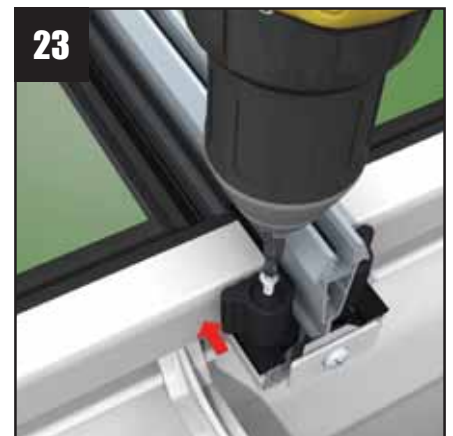
23 Centralise the glazing between the glazing bars. If necessary pack it out on each side - press it down onto the support trim. Using the fixings provided, screw down into the bar as shown.
