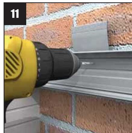
11 Drill through the wallplate main body and directly through each carriage to suit the masonry anchors being used (not supplied). Mark the position of each masonry anchor on the house wall and drill the house wall to suit.
